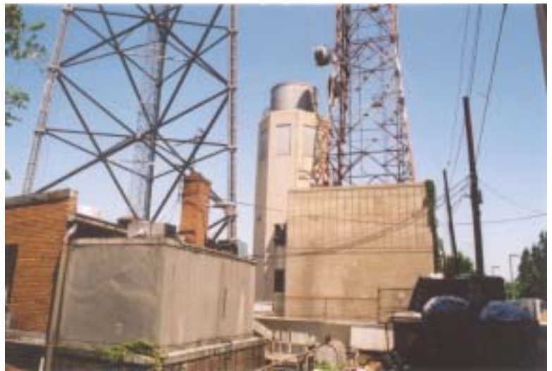
Western Union Tenley Site: American Tower structure (left), Western Union building and tower (right).
