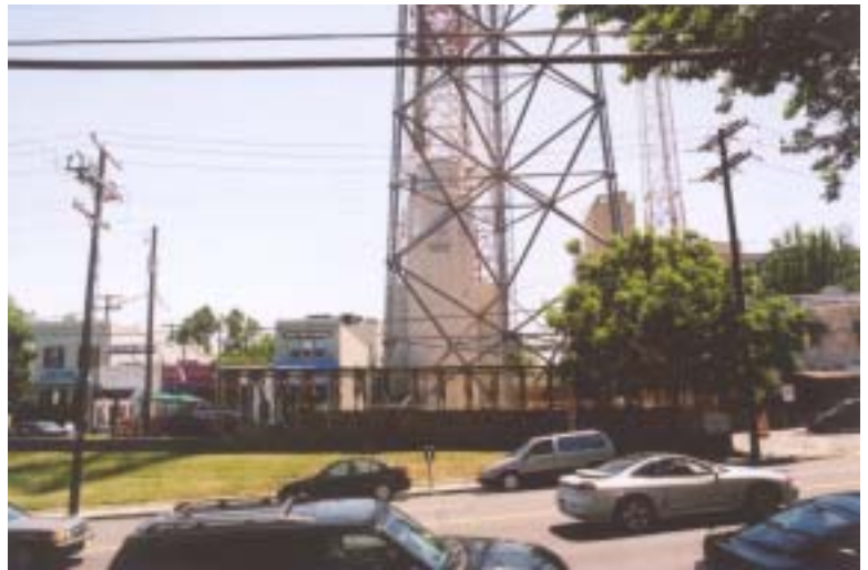
Western Union Tenley Site: American Tower structure in front of building.
