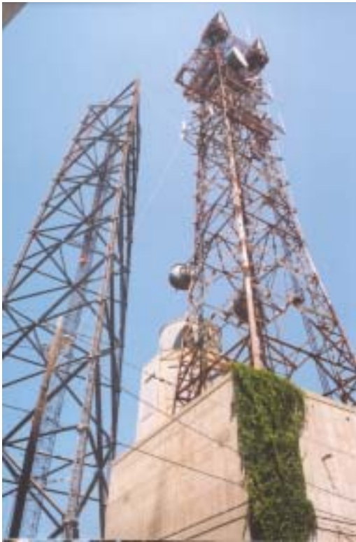
American Tower structure (left), Western Union structures (right).
